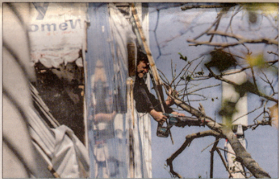
Greg Slattery trims branches from an upper-level window of the 19th-century home "Broadmoor" as it makes its way down Boston Neck Road to its new location near Wood Avenue on Tuesday morning.
